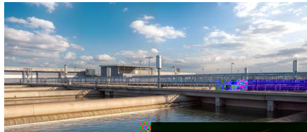
Municipal Water Supply
