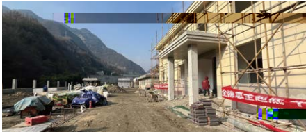
Water Plant Expansion & Upgrades
